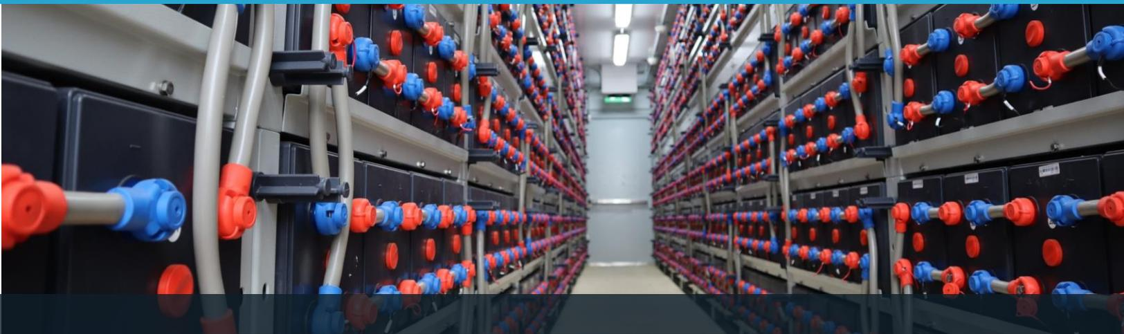
All the battery cells are individually monitored to ensure any deviation in performance is detected and corrected before there is a problem. The battery is operated at partial state-of-charge so that it can accept and deliver charge at all times.
