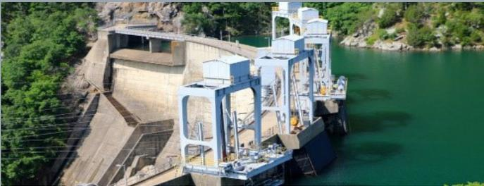
Pumped hydroelectric storage uses electric energy to power pumps that push water up to an elevated retaining pool. When electricity is less abundant and more expensive, the water flows down from its elevated position through a turbine, generating electricity.
