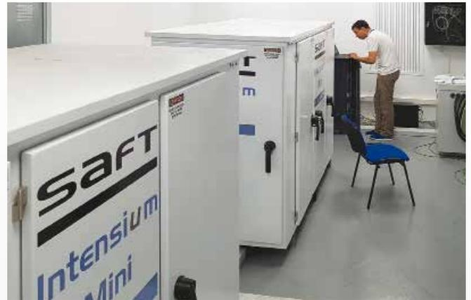
Illustration 4: Saft Intensium® Mini lithium-ion (Li-ion) energy storage systems (ESS) 'behind-the-meter' at EXKAL manufacturing site in Navarra, Spain.
