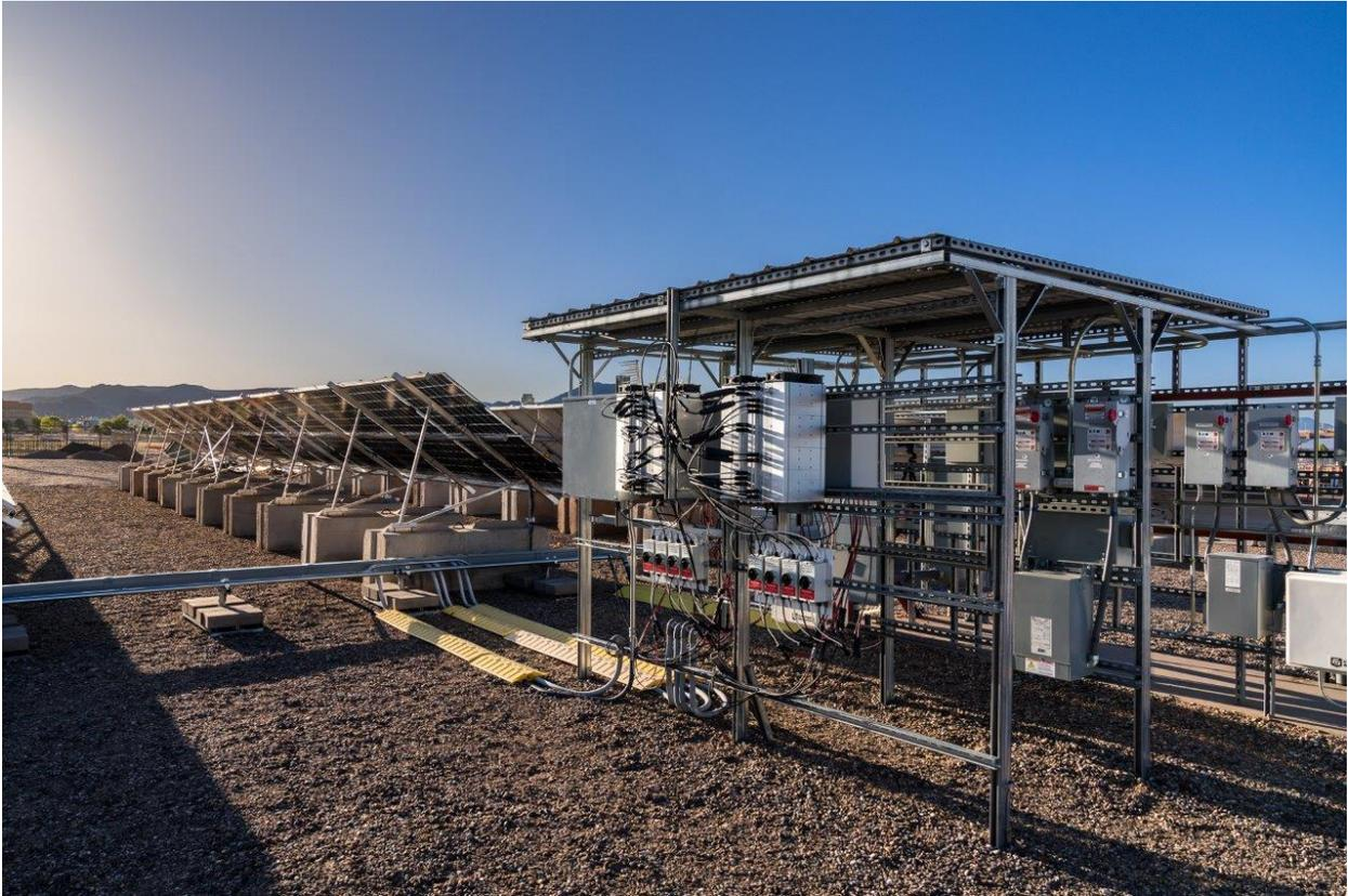
*Figure 3: The Alencon SPOTs serve to harvest power from the central PV arrays in ETL's BlockEnergy Microgrid and deliver a fixed voltage to the DC distribution bus that connects to each of the nano grids. The SPOT's galvanic isolation isolates the grounding of the PV arrays from the DC bus to enable ETL's protection scheme for the Microgrid to assure a high level of safety and resilience.*
